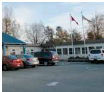
SOUTH POPLAR ELEMENTARY
